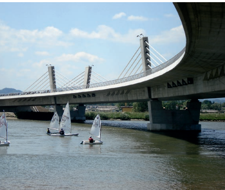
The Puch's bridge in Ptuj.
