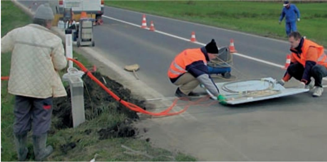
Fig 1: Live road installation of an experimental fibre optic axle detector near Sp. Polskava.
