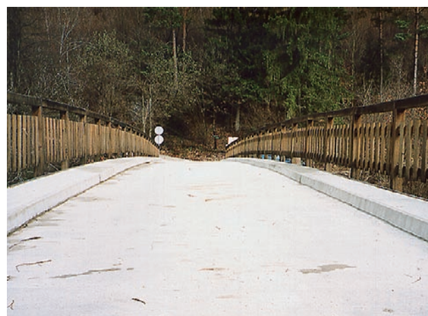
Figure 10: Overlay on the bridge over the Sava Bohinjka River near Mačkovec.
